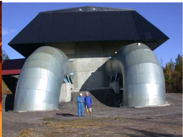
Figure 8. Air intakes for primary shafts (4.5 m diameter)
