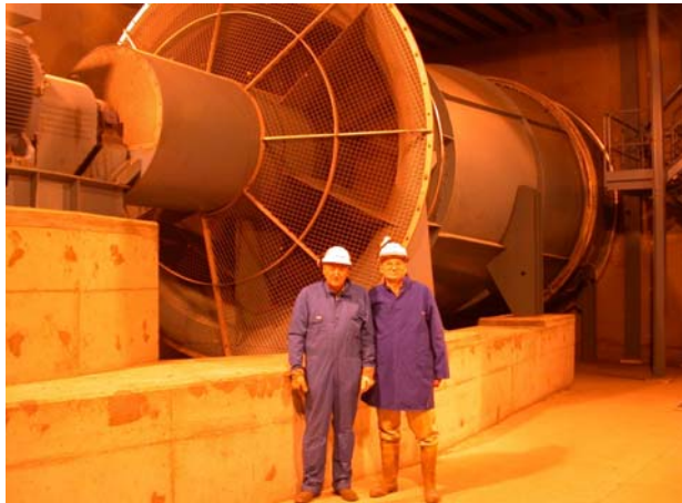
Figure 7. Fan installation at Dennewitz
