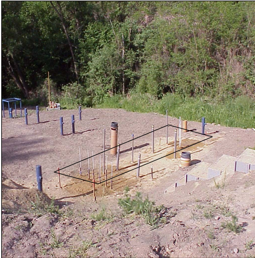
Fig. 14: Position of PRB with monitoring wells
