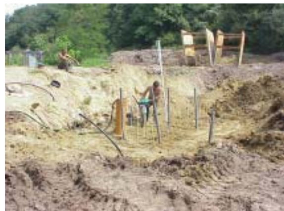
Fig. 3: Construction of the experimental PRB in Pécs, Hungary
