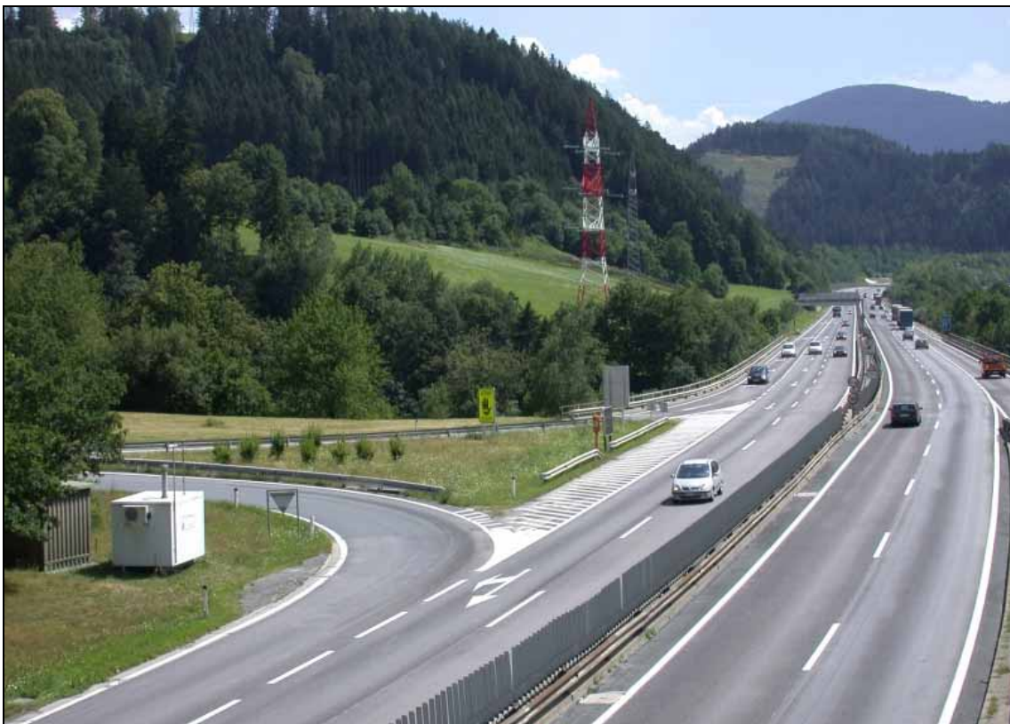
Figure 9: Flat terrain (free air flow) without large buildings and forest up to several tens of metres, Gärberbach A13, Tyrol, Austria (source: Amt der Tiroler Landesregierung).
