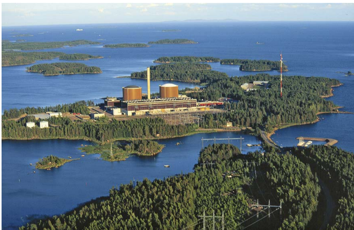
Figure 6-1. The Loviisa power plant is located on Hästholmen island.
