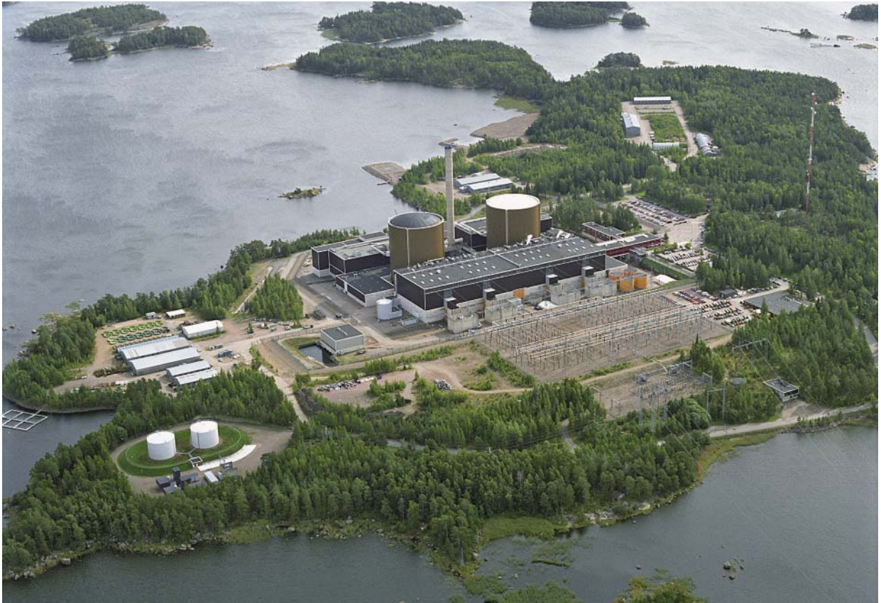
Figure 6-5. An aerial photo of the plant and its surroundings.
