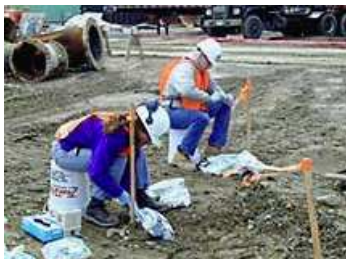
Figure 3.1.4. Collection of soil samples from former Maine Yankee nuclear power plant site 54
