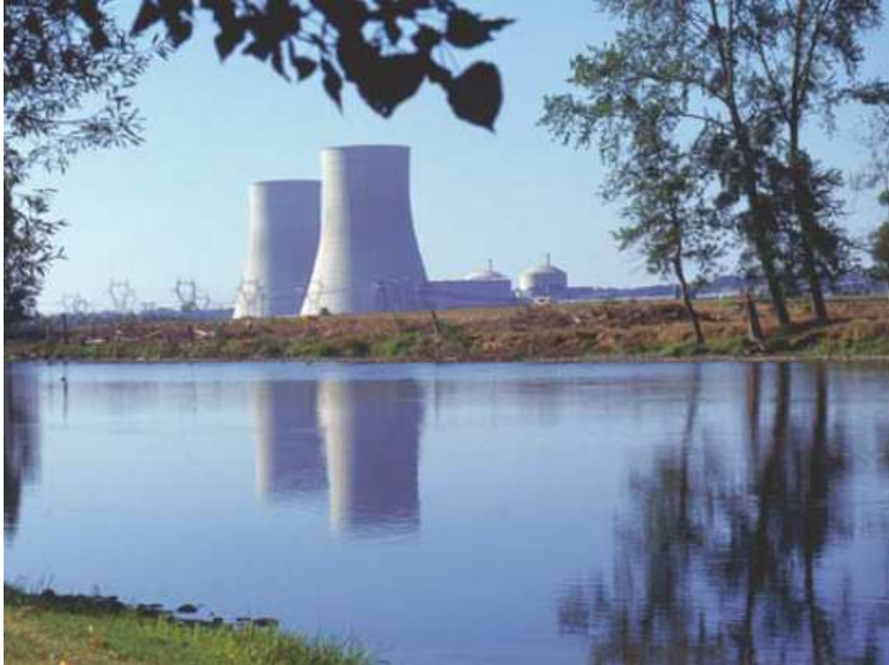
Fig. 4.3.32 Nuclear power plant Civaux 1&2 (France) with wet natural draught cooling tower.
