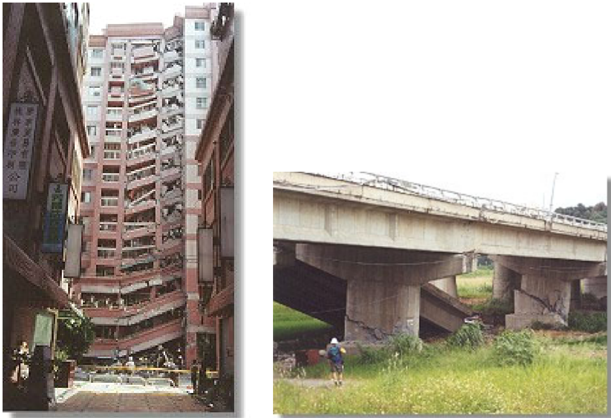
Figure 2.2: Damages due to the Chi-Chi earthquake, Taiwan, September 20, 1999, Magnitude 7.6 [5]
