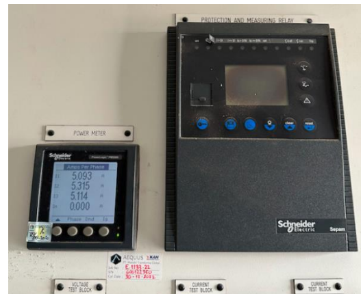
The energy meter (Schneider PM5560 0.2S)
