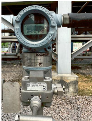
The compact orifice plate flow meter for lean gas (Rosemount 3051CFC)
