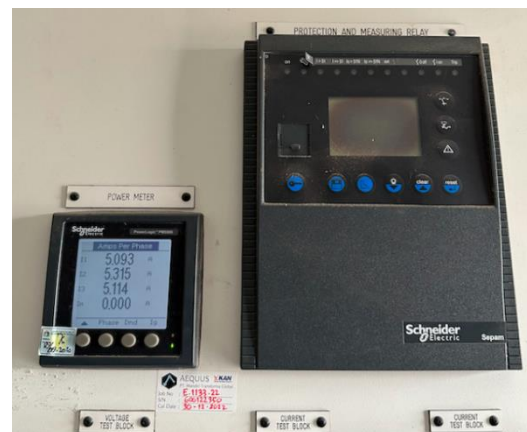
The energy meter (Schneider PM5560 0.2S)
