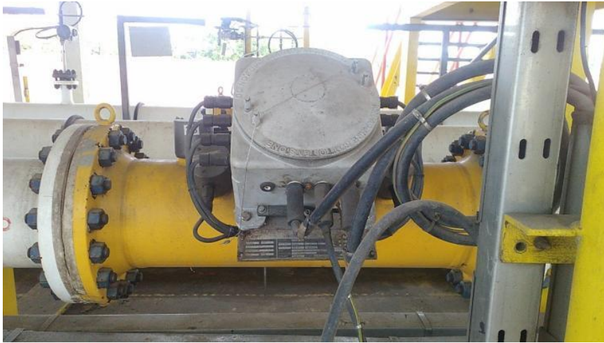
The Ultrasonic flow meter for feed gas/at Point F (Elster Instromed Q. Sonic 4C)
