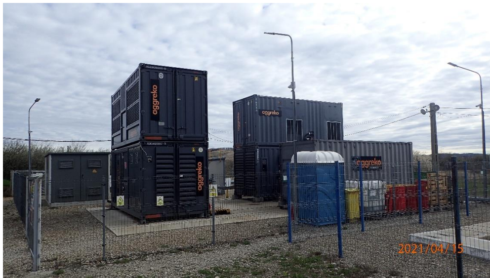
Figure B: The 2 G2P units operated by Aggreko
